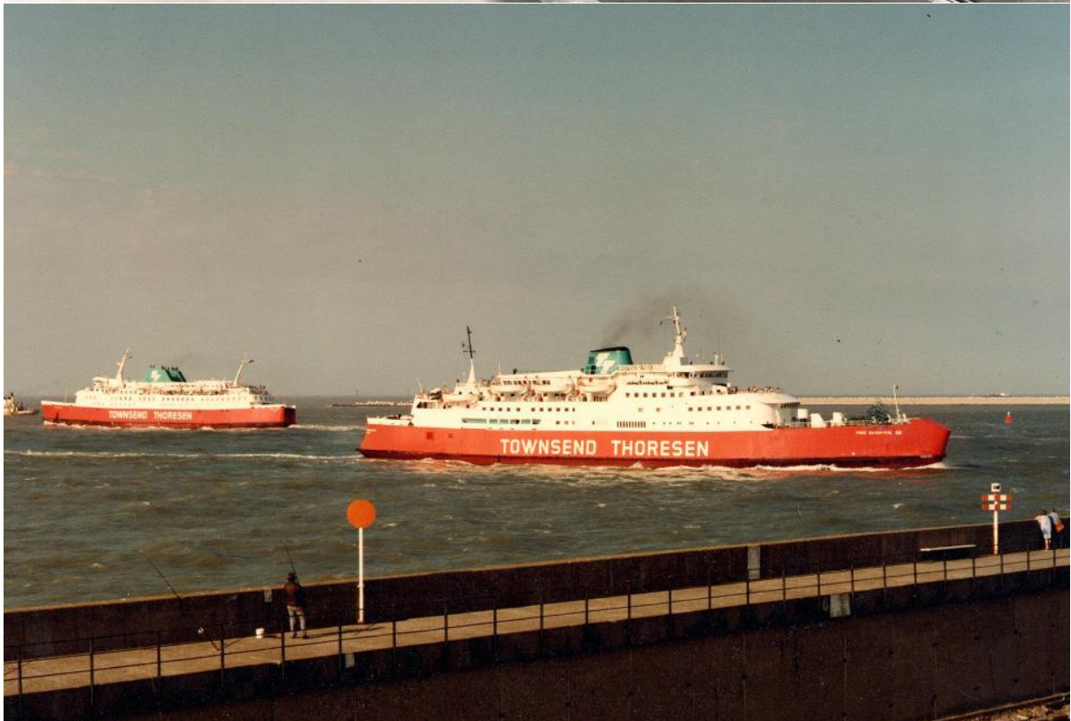
The works for the overall expansion were carried out between 1972 and 1985 and included the construction
