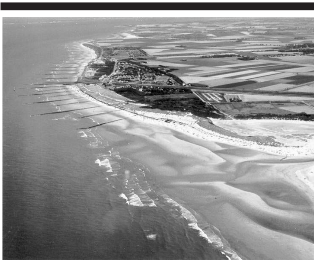
Figure 15. The contemporary Zwin inlet at low tide, seen from the air (photo from a PIANC pedagogical document). Field of groins is on Dutch territory, but another exists also farther south on beach area of Knokke municipality.
